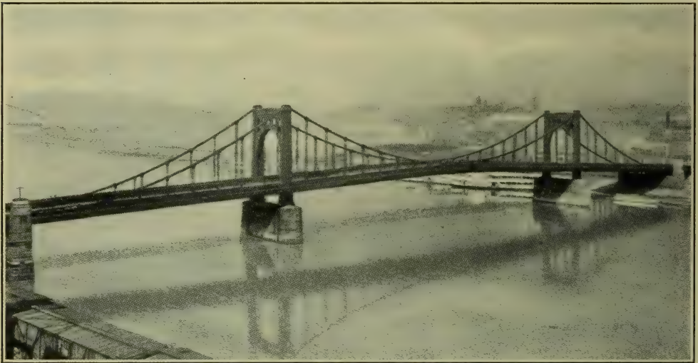
FIG. 13.—The New Sixth Street Chain Bridge over the Allegheny River in Pittsburgh, Pennsylvania, Span 442 feet
